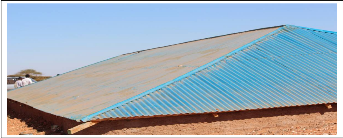
Figure 3: Underground water tank
